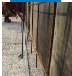
Laying Idrostop B25
