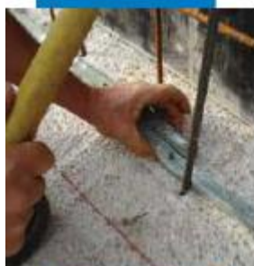
Fixing Idrostop B25 in place
