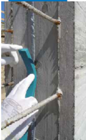
Applying Idrostop Soft on vertical surfaces
