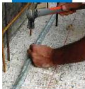
Fixing Idrostop B25 in place
